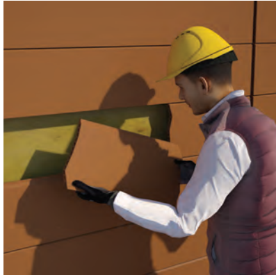
Remove the broken product.
