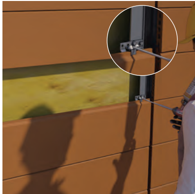
Put dots of glue on the clips (use polyurethane glue type SIKAFLEX 11 FC).
