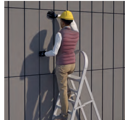
Check the alignment of the installed product and the stability.
