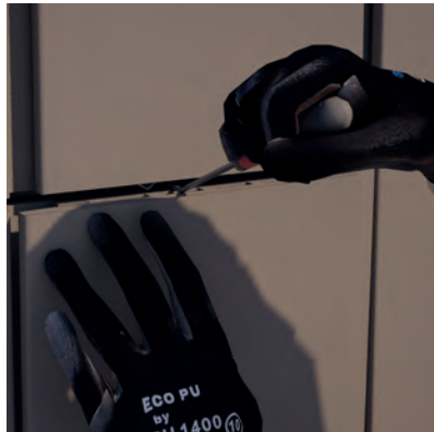
Using a flat screwdriver or similar object (with plastic protection i.e such as electrical tape wrapped onto the flat blade so as not to chip the terracotta), lift each clip one by one to put them on hold on the full edge of the product. Then press on the product to permanently engage the V-clips® in the cells.
