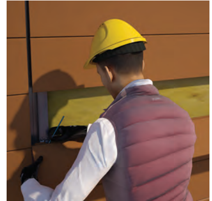
Locate the positioning of the 2 visible standard clips.
