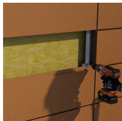
Install the high clip PITA02.
