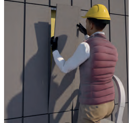
Install the V-clip® on the lower part of the replacement terracotta product. Place the terracotta product by clipping the V-clips® on the bottom rail.
