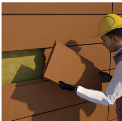
Remove the broken product.
