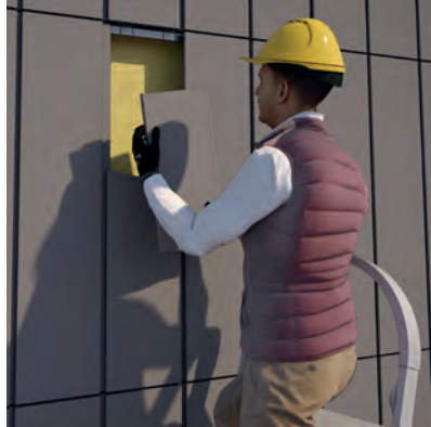
Remove the broken product.
