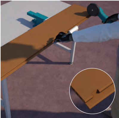
Trace the cutting area on the replacement product. The cutting of the product in the upper part is necessary in order to be able to fit the cut area in the upper clip
