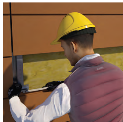
Locate the positioning of the 2 visible common clips.
