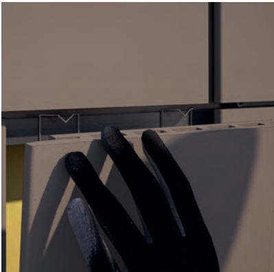
Install the waiting V-clips® on the upper rail, where the cells will be positioned. Make a rocking movement to advance the terracotta product towards the high clips.
