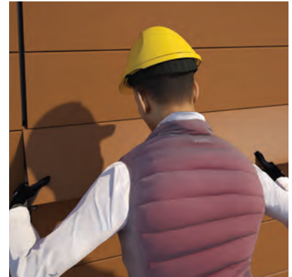
Put the replacement product in place by first inserting the upper part, pushing towards the wall then exerting downward pressure to position it at the bottom of the clips.
